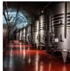
INDUSTRIAL ENERGY AUDITS
